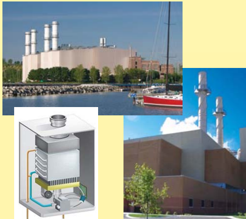
Highly Efficient Natural Gas Combined Cycle Power Plant (TOP), Natural Gas Cogeneration Plant (RIGHT), Tankless Water Heater (LEFT)
