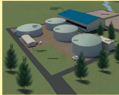
Community Manure Digester in Dane County Wisconsin: Two large and one medium-sized dairy, 2 MW of electricity and phosphorus removal system
