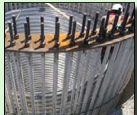
20 foot long bolts attach the turbine to the foundation
