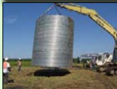
The inner cylinder arrives and is lowered to the ground
